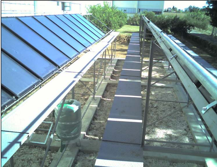
The platform and its concrete foundation
